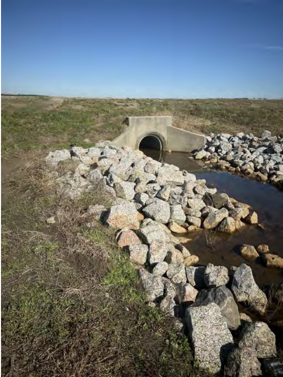
Culvert – Facing North
