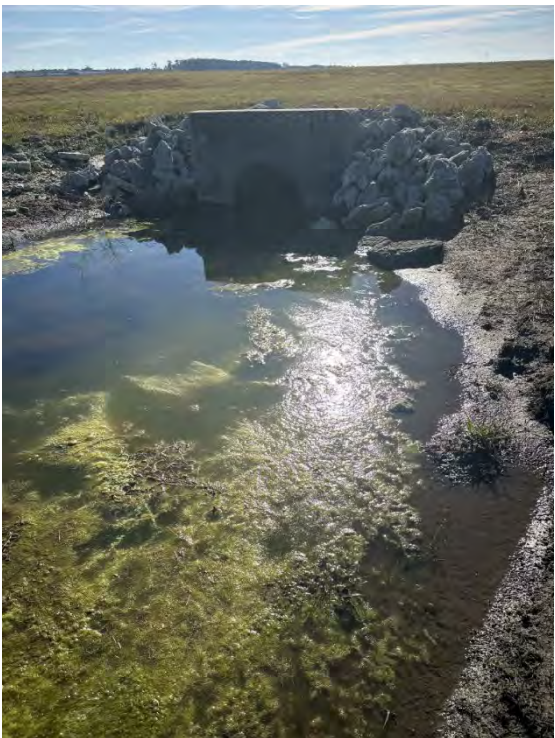
Culvert – Facing South
