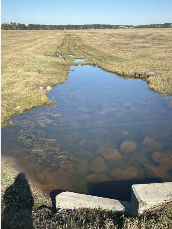
Above culvert – Facing North
