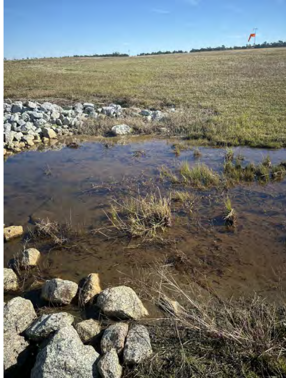
Water depth ~3" – Facing East
