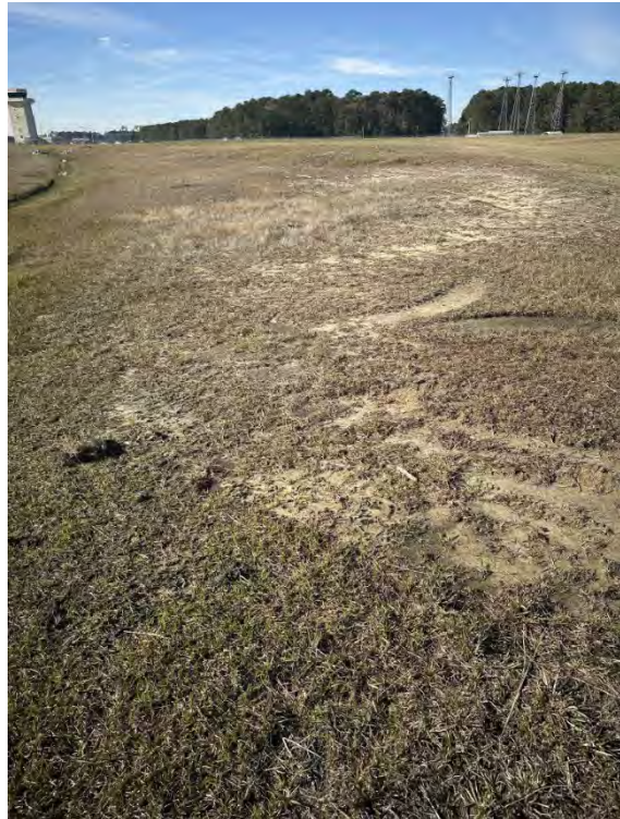
Typical Condition – Facing West
