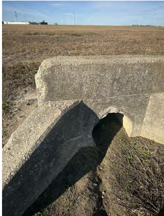
Dry culvert – Facing West
