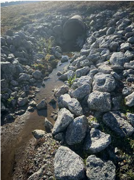
Culvert; water depth ~ 1-3" – Facing South
