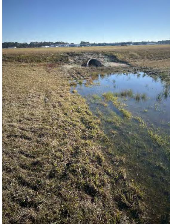
Culvert – Facing East
