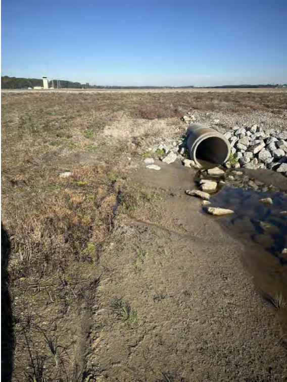
Culvert– Facing North
