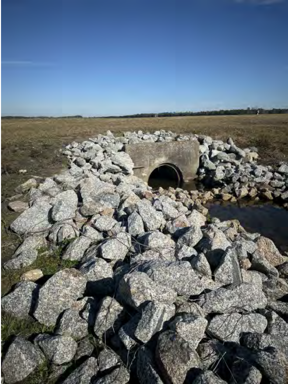
Culvert – Facing North
