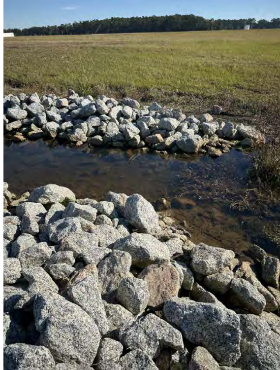
Typical Condition – Facing East
