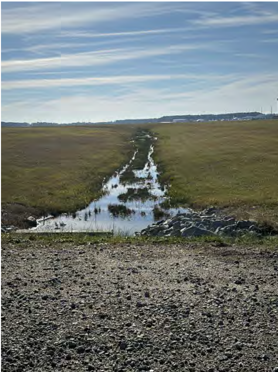
Typical Condition – Facing South
