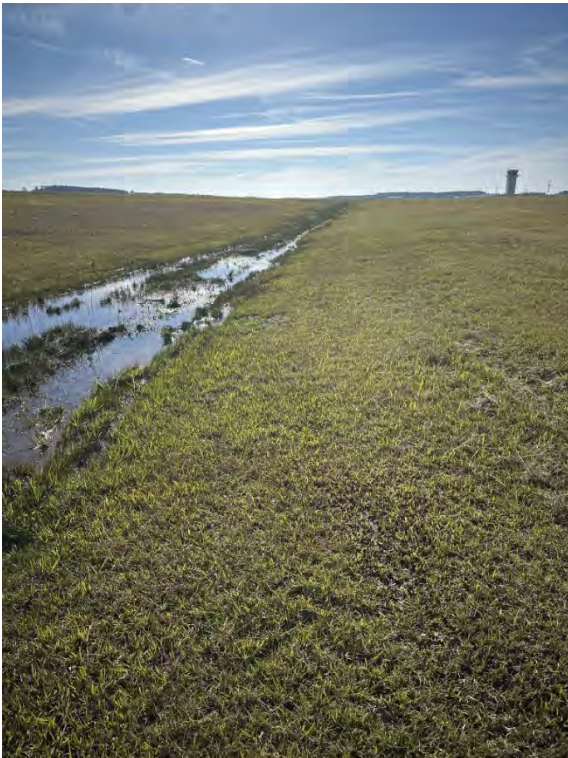
Typical Condition – Facing South
