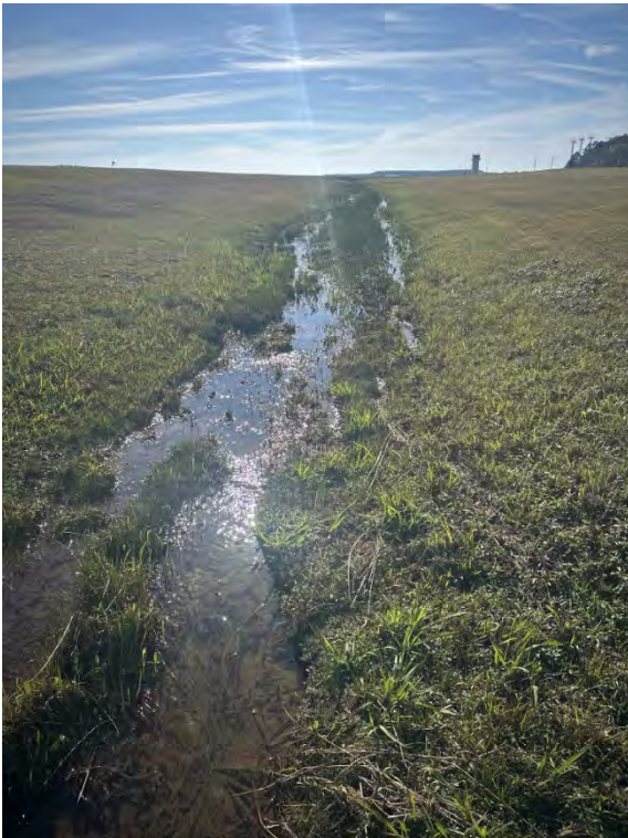
Typical Condition – Facing South
