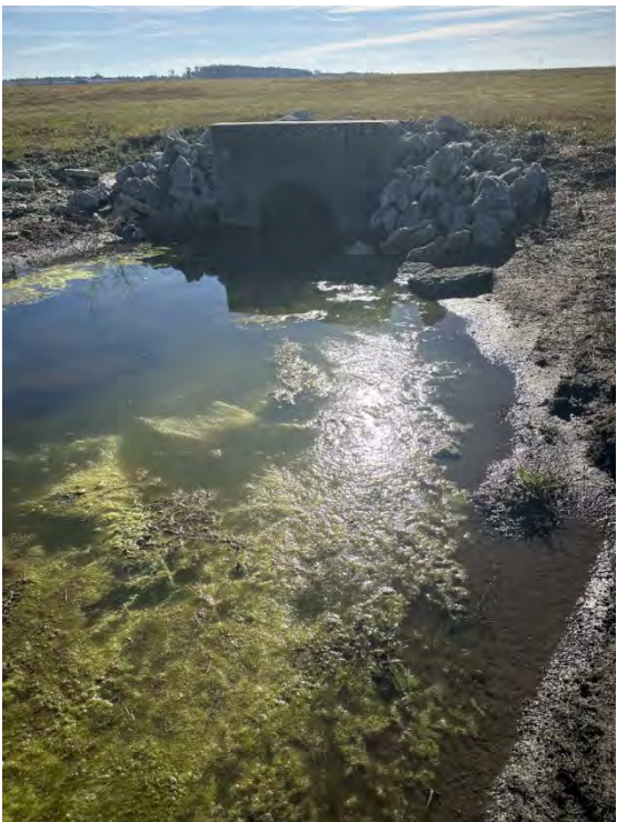
Culvert – Facing South
