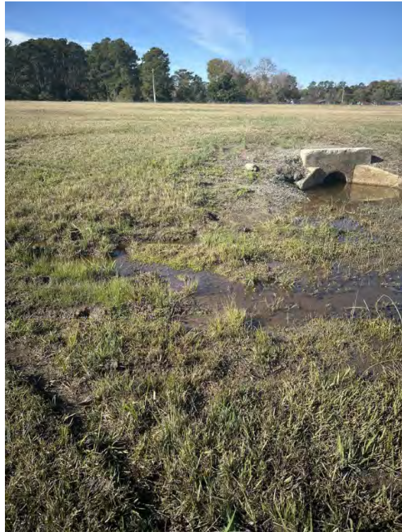
Culvert – Facing West
