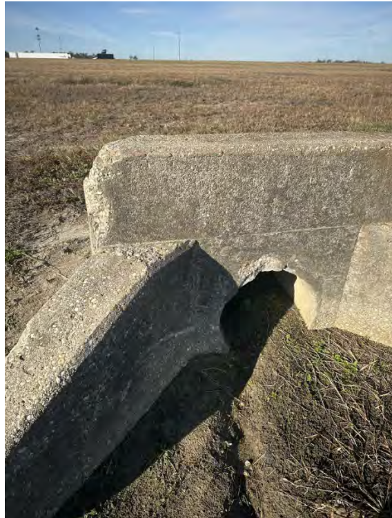
Dry culvert – Facing West
