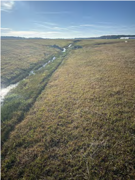
Typical Condition – Facing South
