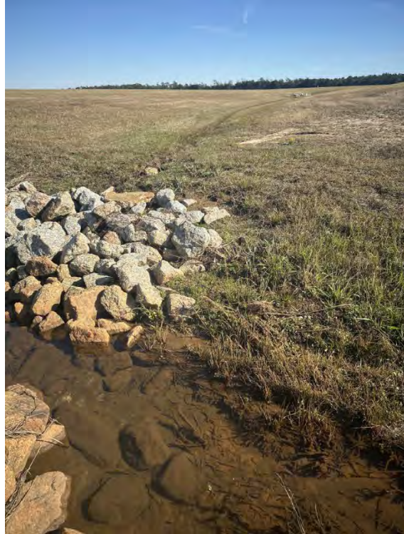
Typical Condition – Facing East
