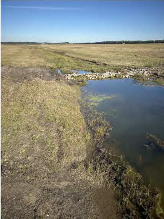
Culvert – Facing North
