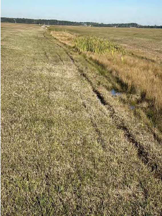
Typical condition – Facing North
