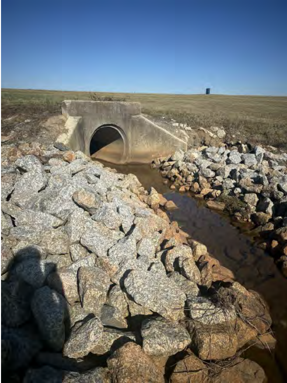
Culvert – Facing North
