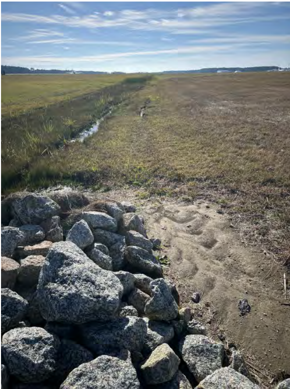
Typical Condition – Facing South
